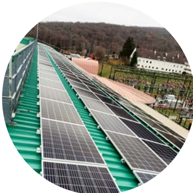
ELECTRICITY-GENERATING frequency inverter in Auhof, Vienna
