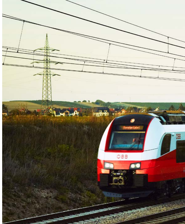
BRANCH LINES. Branch lines in the ÖBB network will be electrified step by
