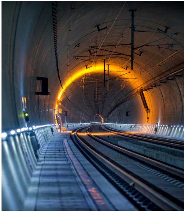
TOP OF THE LINE. Catenaries are obviously standard in the new tunnels on high-speed lines
