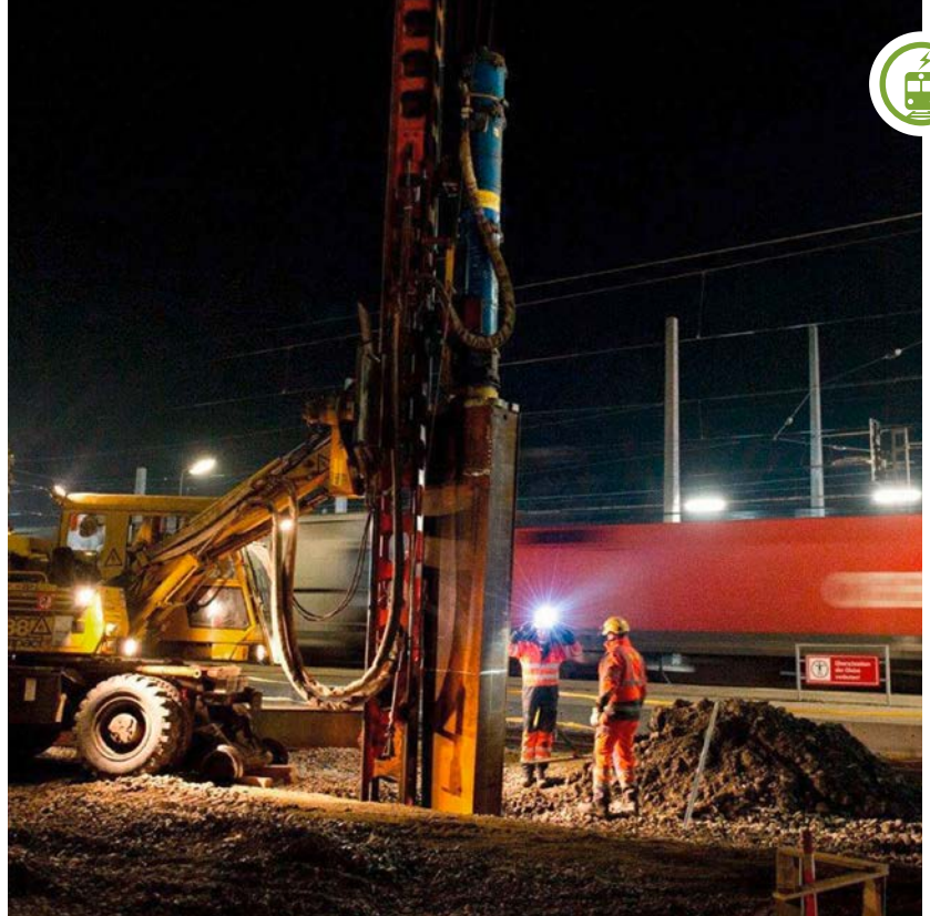
CATENARY MASTS are rammed into the ground by machine
